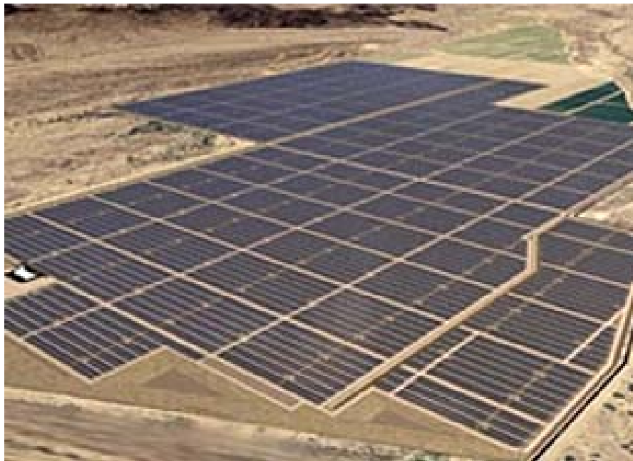
Figure 1.8: Large solar PV fields in operation today [27]
