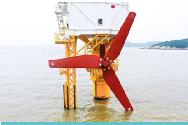
Offshore Step-up Station and 300 kW Turbine
