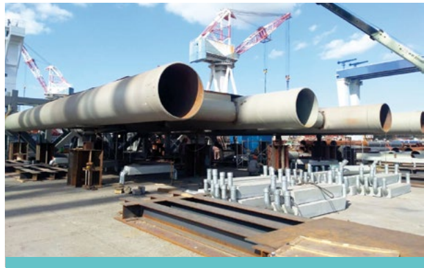
#2 platform assembled at the dock
