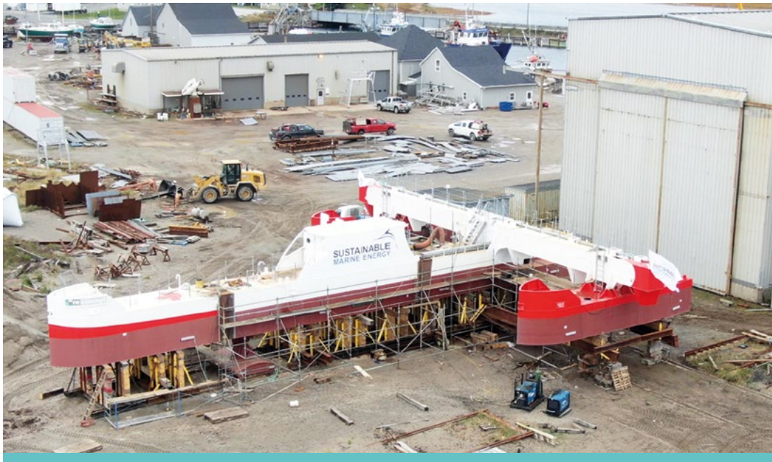
Construction of Sustainable Marine's 420 kW PLAT-I platform
