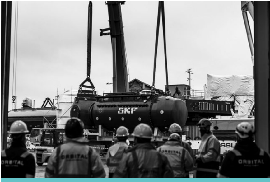
Power train for Orbital Marine Power's O2-2000, developed and manufactured by SKF
