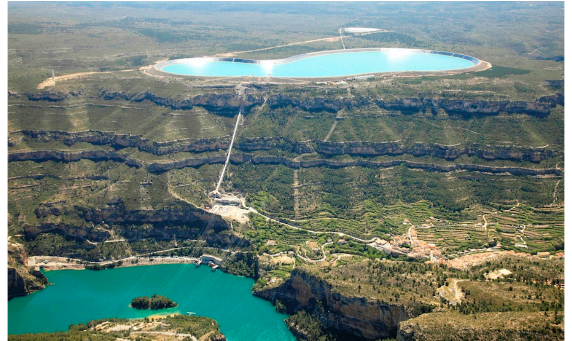
Bath County PHS plant, commercial operation since 1985. Picture source : www.enr.com
