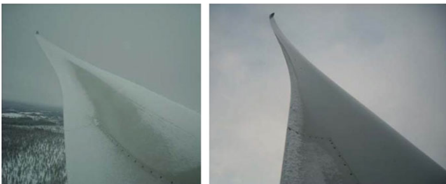
Fig. 5.17 Picture of a Enercon E82 blade with de-icing on (left) and off (right) [17]
