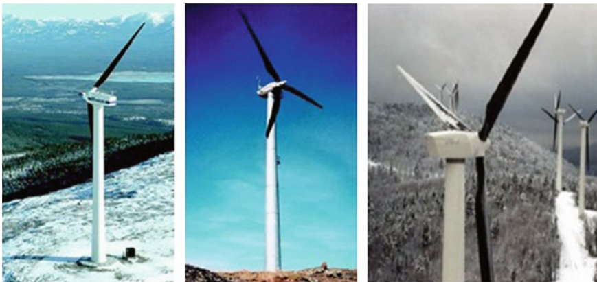
Fig. 5.6 Vestas V47-660 ( left ) and Bonus 150 kW ( centre ) with black-painted fluorourethane (Sta-Clean) coating. Searsburg turbines ( right ) with black paint applied to the blades: note the layer of ice along the blade leading edge (Color figure online)
