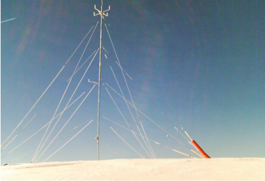
Fig. 2.23 Image of the iced met mast
