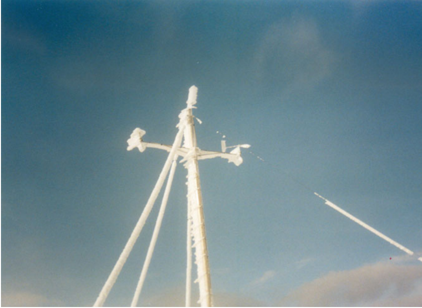
Fig. 2.26 Severe icing of an anemometer and wind vane
