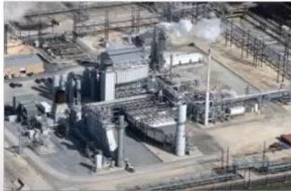
The Air Products and Chemicals hydrogen production facilities in Port Arthur, Texas, is funded by the Energy Department through the 2009 Recovery Act. | Photo credit Air Products and Chemicals hydrogen production facilities.
