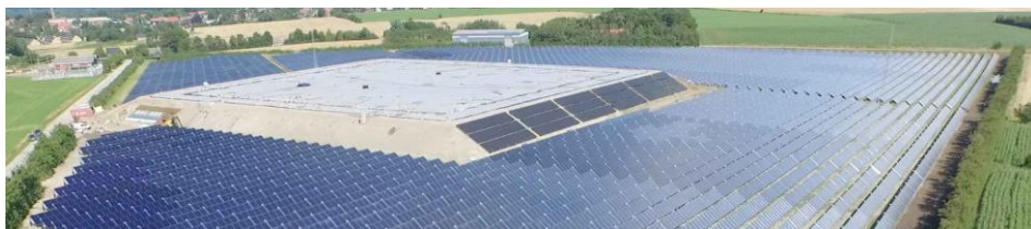
Figure 12 Solar field and seasonal storage pit of Gram's DH system (Source: Gram Fjernvarme)
