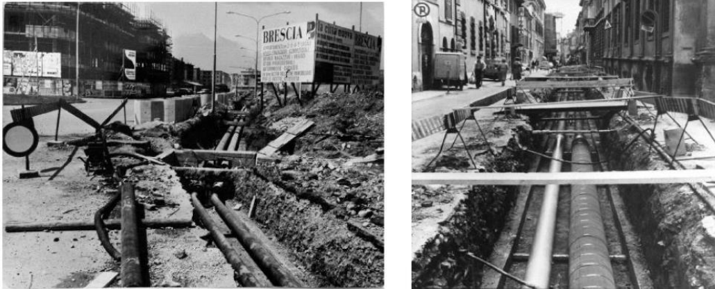
1972 – Realization of DH network in Brescia 2 area Early '80s – Realization of DH network in city center
