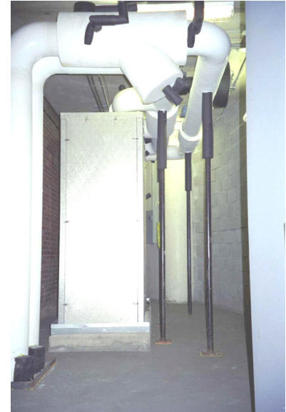
Part I Figure 7.3: ETS after installation
