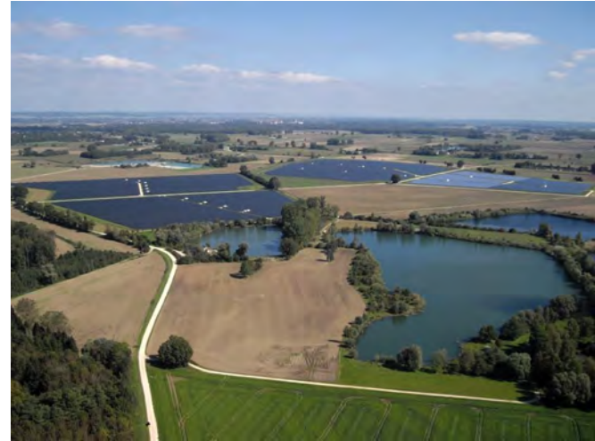
Figure 15.3: The 25.7 MW p Lauingen Energy Park in Bavarian Swabia, Germany [82].
