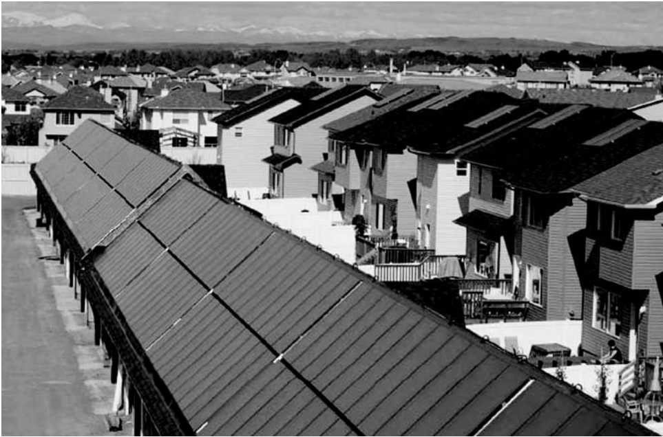
Figure 8.32 Photograph of one row of houses and garages covered with solar collectors in the DLSC (Courtesy of DLSC). Source: “The Drake Landing Solar Community Project – Early Results.” B. Sibbitt, T. Onno, D. McClenahan, J. Thorton, A. Brunger, J. Kokko, B. Wong, Natural Resources Canada, 2007. Reproduced with the permission of the Minister of Natural Resources Canada, 2010
