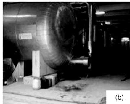
Figure 8.23 (a) The Bangsar district cooling plant and (b) the STL system (Courtesy of Cristopia Energy Systems)
