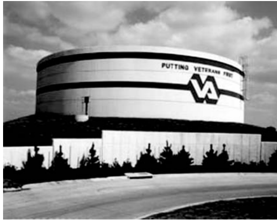
Figure 8.18 The VA Medical Center's 12,491 m 3 stratified water storage tank (DOE, 1999)
