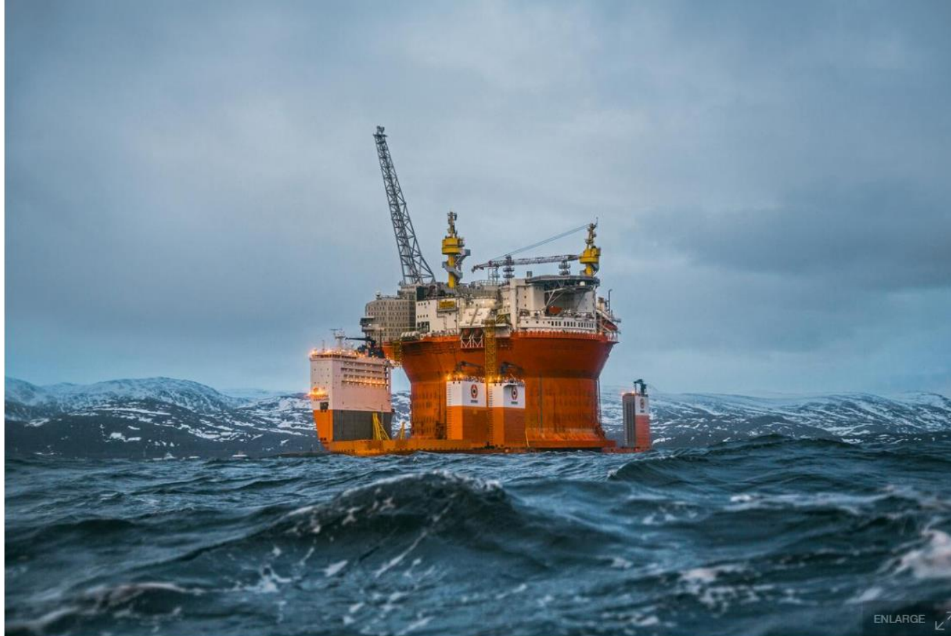
The new Goliat platform awaits commissioning in a fjord near Hammerfest, Norway, last April. Now moored in the Barents Sea at 71° north, it's the world's northernmost offshore oil platform.
