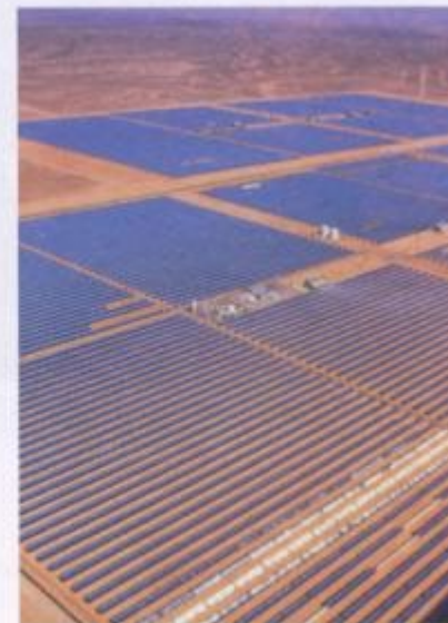
Figure 2.45 SEGS solar collector field – aerial view
