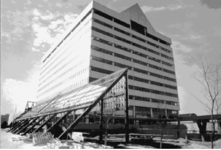
Figure 1. Scarborough Town Centre: first building ATES combined heating and cooling in Canada.
