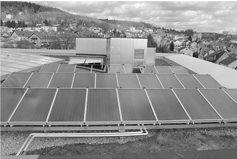
Figure 273. 70 \text{m}^2 collector array, in the background: casing of dehumidifier and regenerator
