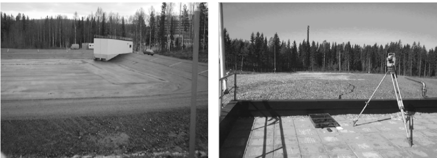
Figure 203. Right: Part of the snow pond with pump house and half of the hospital. Left: Snow covered with wood chips in beginning of the cooling season. Picture taken from the pump house
